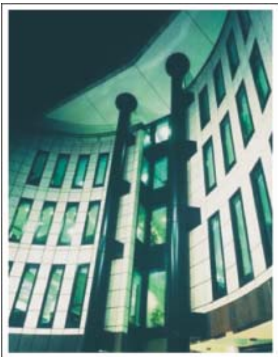
Freshfields Offices - UK
